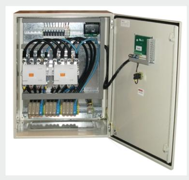
Cubicle composed of the electronic control module which is detecting a mains failure and of 2 contactors mechanically and electrically interlocked or a motorized switch controlled by the above electronic controller who are realizing the change of supply from the GEN SET or the MAINS to the load.
